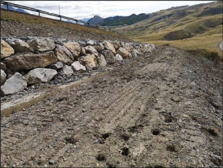
Installation securing a road from landslides
